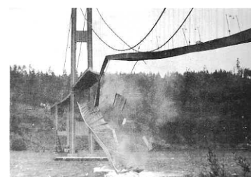
fig 3 Tacoma Bridge disaster
