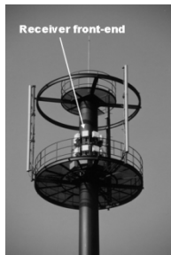
Fig.1. Example of tower-mounted RFE
